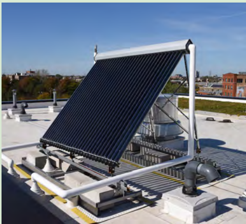
Solar Panel on roof.
