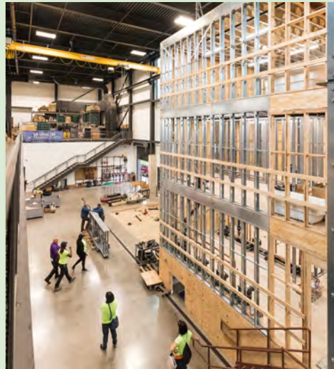
3-story plumbing house.
