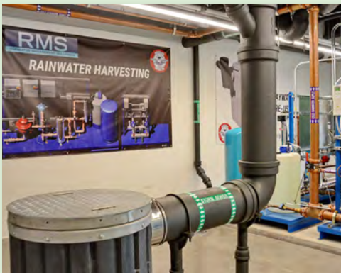
Rainwater Harvesting room.
