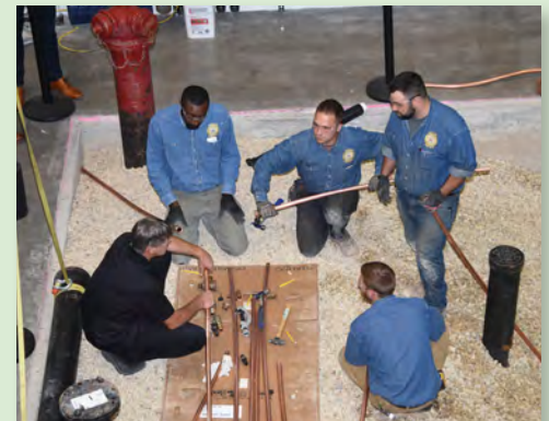
Underground pit (taken from above men working).
